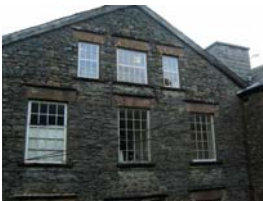
Bainside Studio (top floor)
