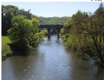
Canal bridge - near where Tarka was born
